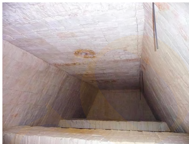
Fig. 3. Pyro-Bloc RTO lining
