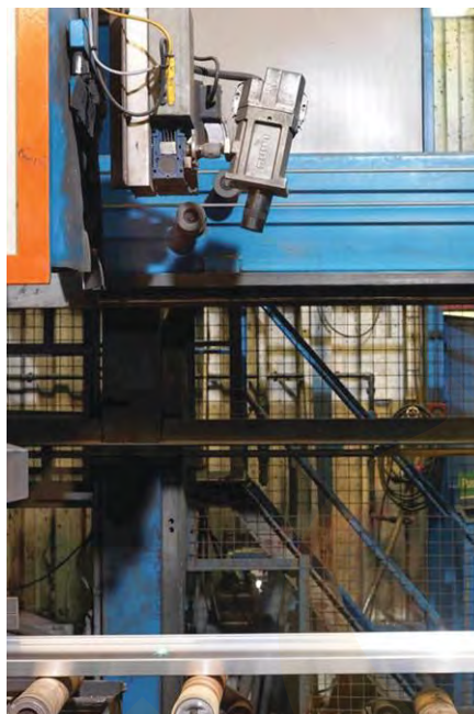
Fig. 6. SPOT AL EQS at the exit of the quench
