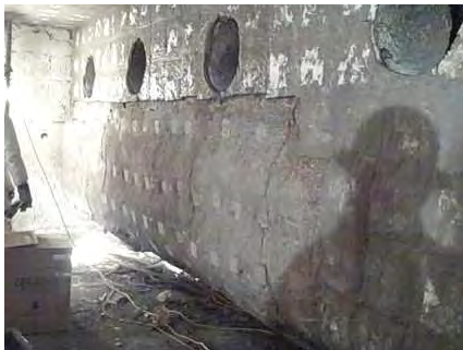
Fig. 1. Spraying bullnose with ITC coating
