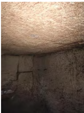
Fig. 7. Soak-zone roof and sidewall
