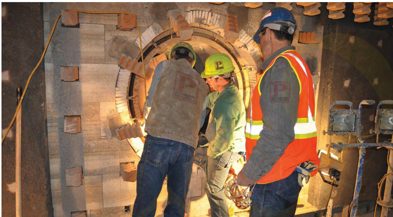
Fig. 1. During the inspection process, the refractory team will provide a comprehensive condition assessment to help determine the need for repair.
