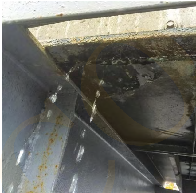
Metal cooling towers are under constant attack by salt air or the caustic atmosphere of many industrial sites. Minerals in hard water as well as its pH level also can contribute to corrosion.
