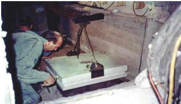
Fig. 1. Installation of ceramic tiles in hearth
